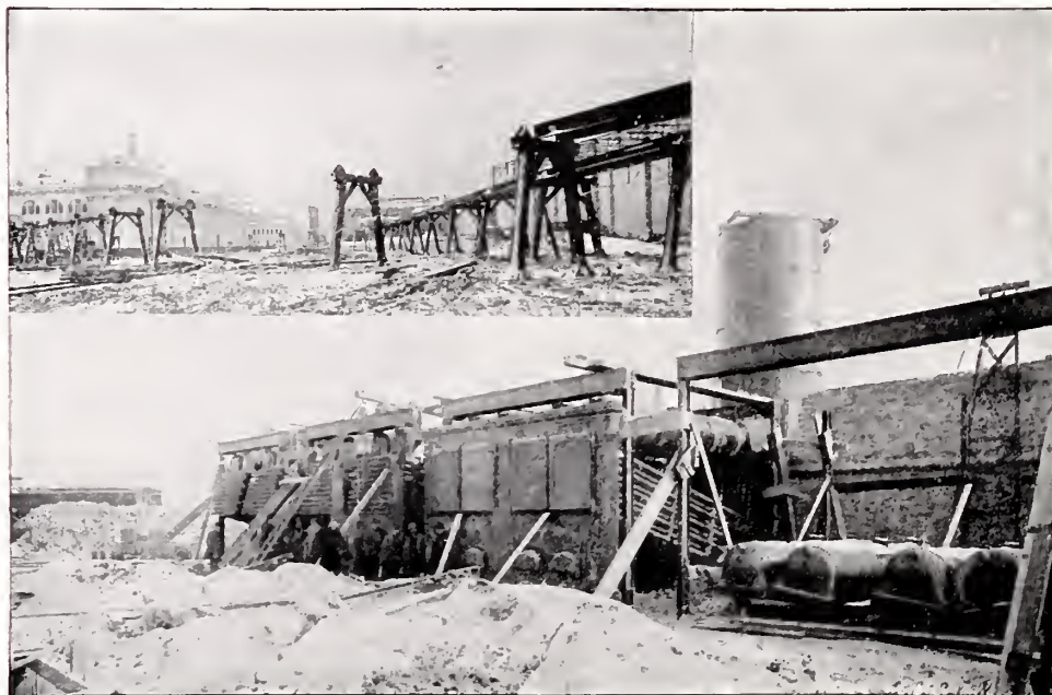
Power House of Intramural Railway at the World's Columbian Exhibition, Chicago, in process of construction, with 5,000 H. P. of Babcock & Wilcox Boilers, 1893.
